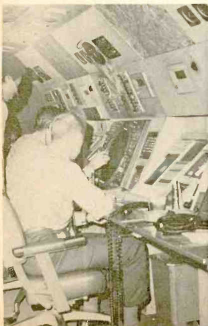
THIS RADAR will not net you a traffic ticket . . . It guides your plane to a safe landing. FAA Approach Radar Control, Douglas Municipal Airport, Charlotte, N. C.
